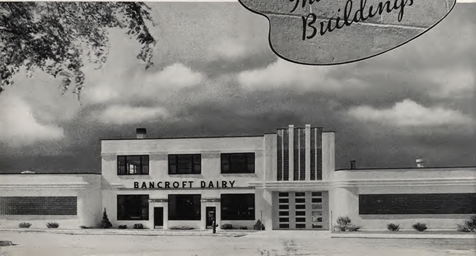
Below —Sanitation and efficiency are “written all over” this modern home of Bancroft Dairy, Madison, Wisconsin. Concrete masonry finished with portland cement stucco resulted in a pleasing appearance at low cost. Law, Law and Potter, architects. Fritz Construction Co., contractor.
